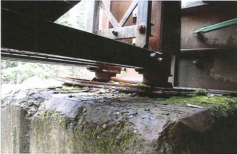
CK2287 Left Abutment bearing plate
