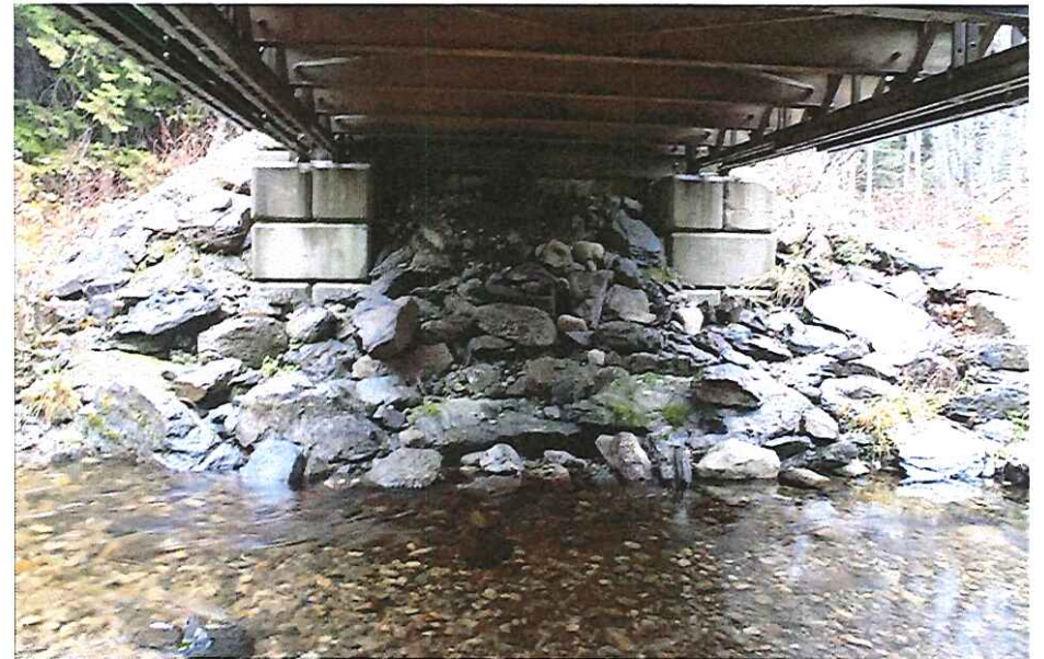
CK2287 Right Abutment
